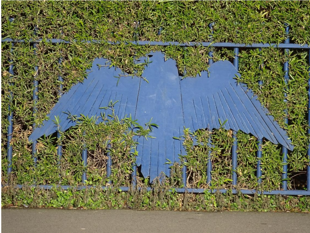
New falcon railings at the site of the former Falcon Works
